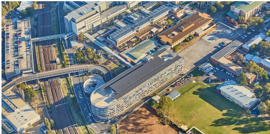
Clean energy: solar panels installed on Liverpool Hospital car park roof
