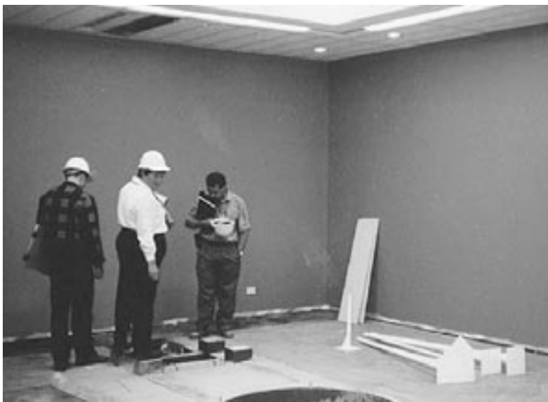
Building the LCTC Radiotherapy Bunker.
