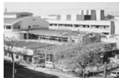
Liverpool Cancer Therapy Centre in various stages through the building process.
