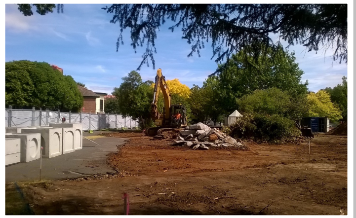
New Mona Road car park construction
