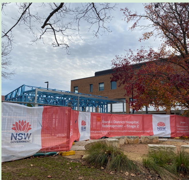
(Top) Concept design and (Bottom) construction has commenced.
