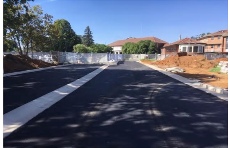
NEW driveway and future parking on the left.
