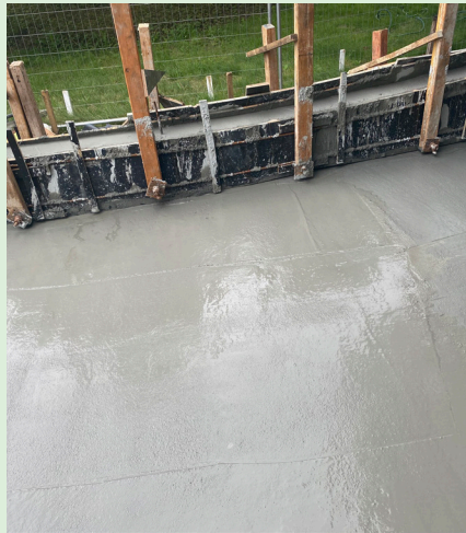
The first concrete pour has been completed for the ramped access to The OC
