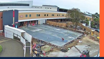
More than 150 cubic metres of concrete was brought into the site for the 600 square metre slab
